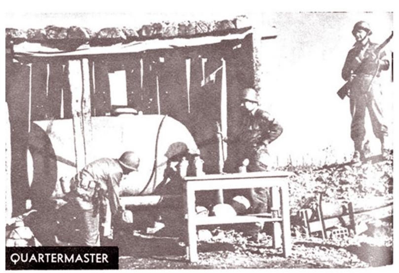
THE QUARTERMASTER CORPS studies this picture of a water supply tank captured by U.S. Rangers in French North Africa, and learns the enemy's methods of construction and use. If details suggest improvements for our own tanks, they will quickly be adapted. Heavy timbers guard it against shrapnel
