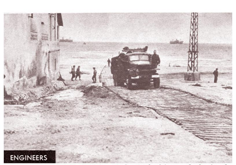
BRINGING THIS 10-WHEEL TRUCK from the landing boat (seen on horizon) and across the sandy beach to solid ground, was an engineering feat. It was accomplished by use of the portable road made of steel mesh which distributes weight, prevents bogging down. Picture may suggest improvements.
