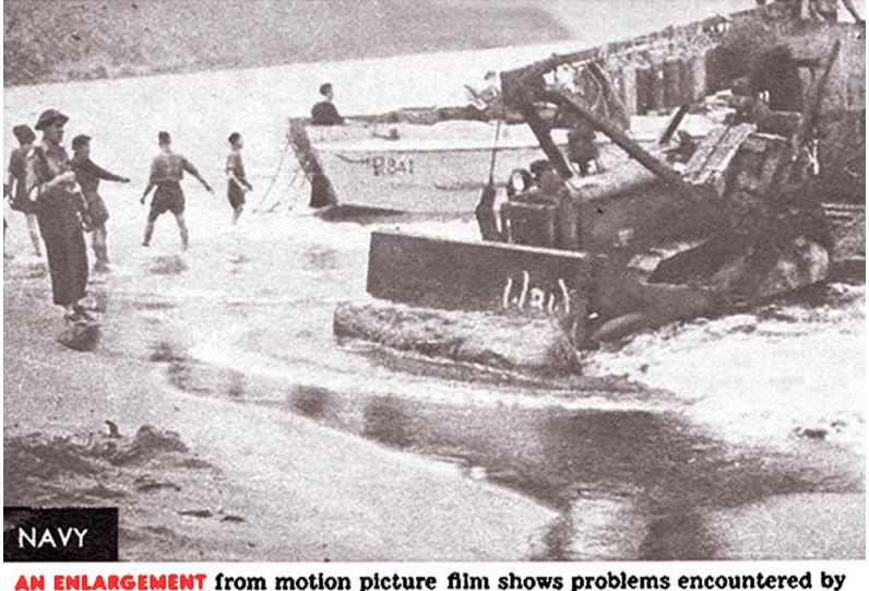
the Navy and by Army Engineers in landing a road-building tractor on the coast of Algeria. New methods of transport are constantly being worked out as a result of Signal Corps' inclusive film record of land and sea operations.
