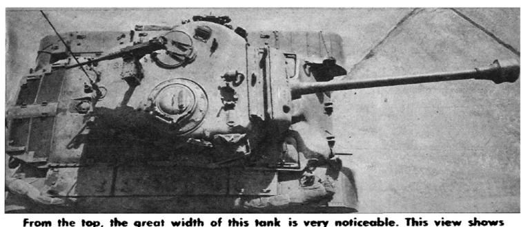
From the top, the great width of this tank is very noticeable. This view shows the triangular shape of the cast turret and the tank commander's cupola.
