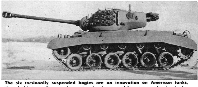
though this type of suspension system has been used for years on foreign tanks.
