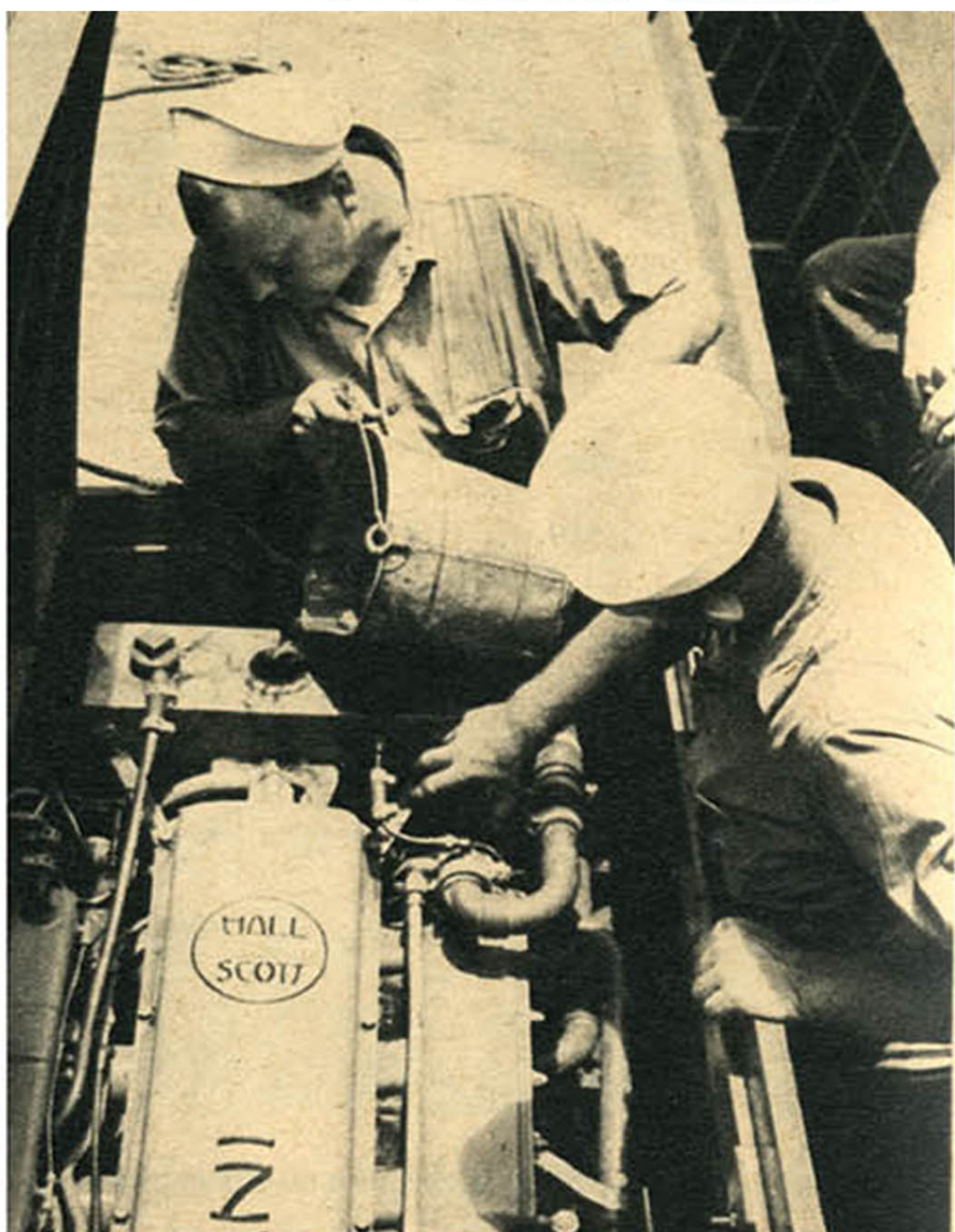
EACH STUDENT IS TRAINED as both engineer and coxswain so one can assist the other in emergencies. This seaman putting water in high-powered Hall-Scott engine will make practice landings, learn practical navigation not in books.
