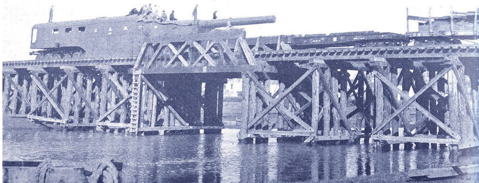
Trestles had to be strengthened to carry the immense weight—275 tons each—of the gun cars as they left St. Nazaire
