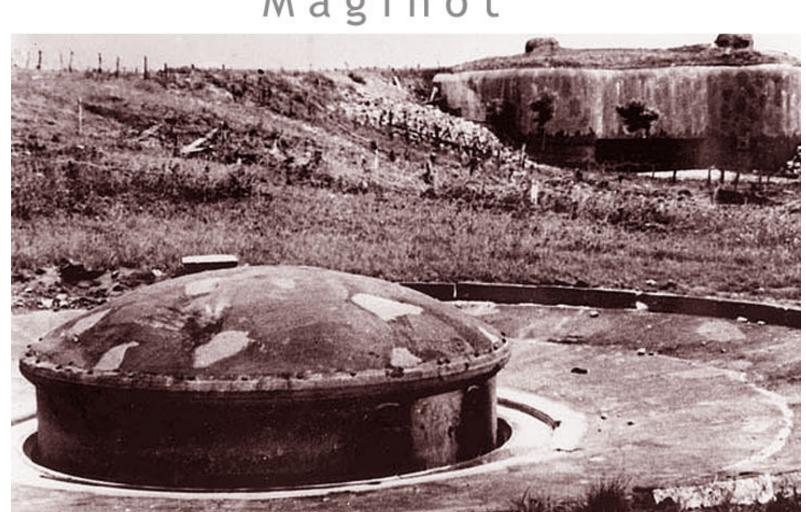
The obtruding pillboxes are of a rotating type. There is no above-ground entrance or exit. Each has two stories—one above ground and the other sixty feet below. Above the lower chamber there is at least forty feet of concrete.
